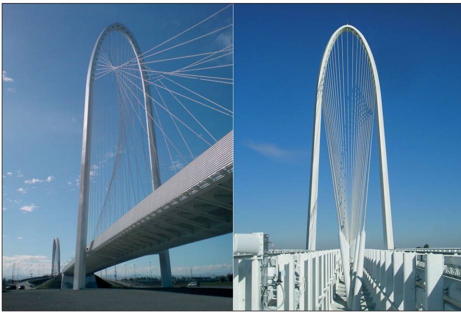
Fig. 3: General views of one of the twin bridges across the roundabouts
