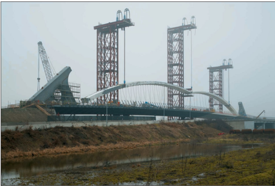
Fig. 5: Erection of the central bridge
